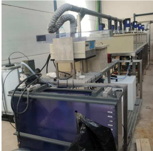
Zinc SX circuit
